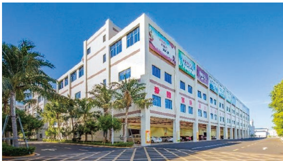
New Hainan Carrianna food factory located at Yunlong High-and-new-tech Industrial Zone in Haikou City
