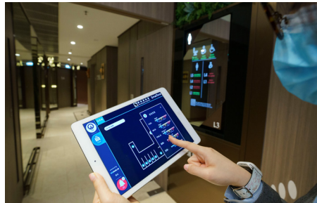
• 5G Smart Restrooms are equipped with sensors to monitor indoor air quality
