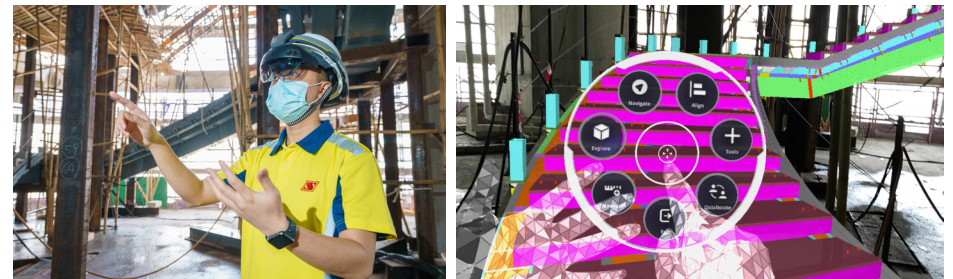
• The Use of MR technology at the construction site
