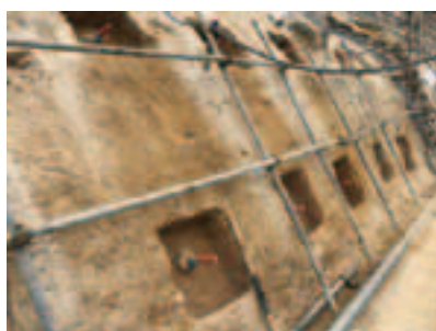
Drilling and installation of soil nails
