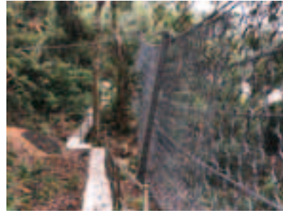
Construction of flexible barrier system
