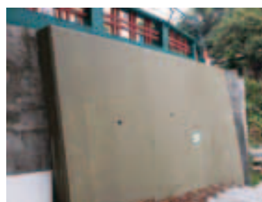
Construction of retaining walls
