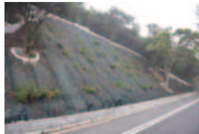
Installation of wire meshes and mats for erosion control
