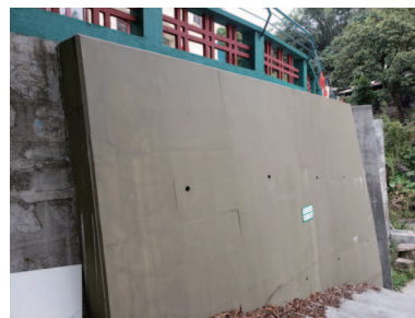
Construction of retaining walls
