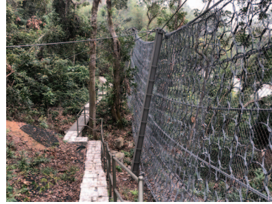
Construction of flexible barrier system
