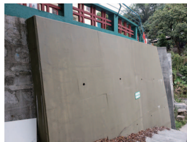
Construction of retaining walls
