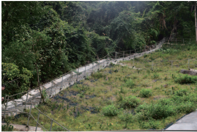
Construction of concrete maintenance stairway/access
