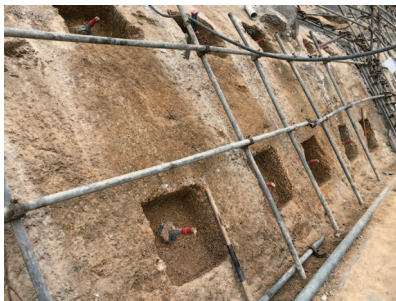
Drilling and installation of soil nails
