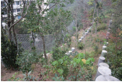
Installation of debris flow protection rigid barriers
