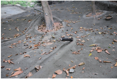
Installation of raking drains
