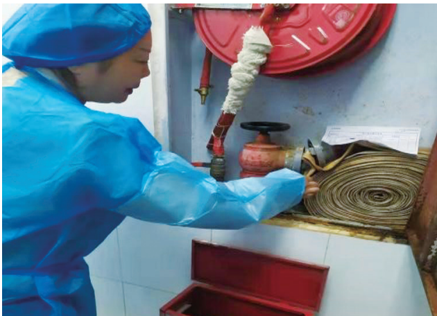
Picture: fire safety inspection
