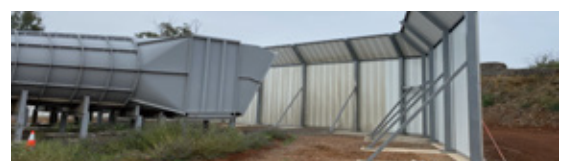
At NPM, a range of noise reduction strategies were used, including the installation of an acoustic wall.
