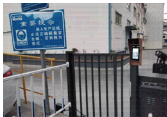
The entrance to our tungsten company has installed an automatic helmet detection system which prevents employees without a helmet from accessing the premises.
