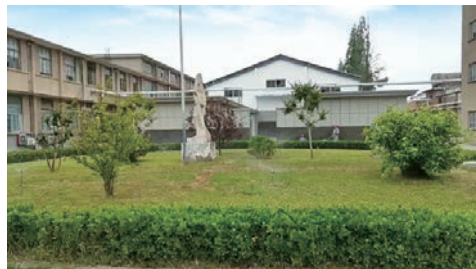
3. The water after sedimentation is used for greening spray in the factory area and as a backup water source for fire fighting
