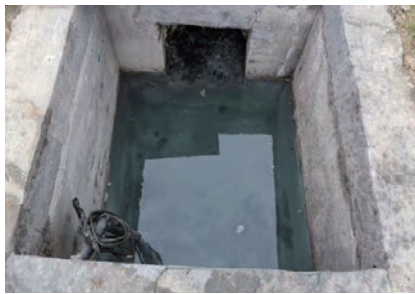
1. Building a wastewater collection tank at the drainage
