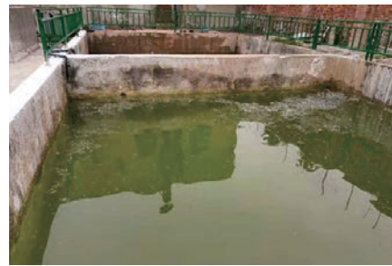
2. Diverting water into the lime pool for exhaust gas from the original boiler for biochemical and sedimentation
