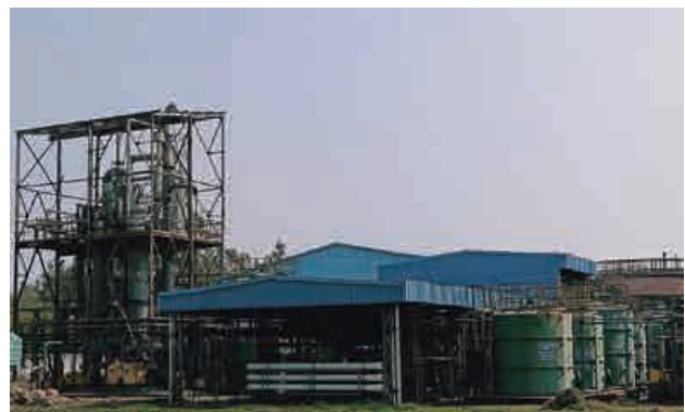
ZLD units in three of our breweries in India.
