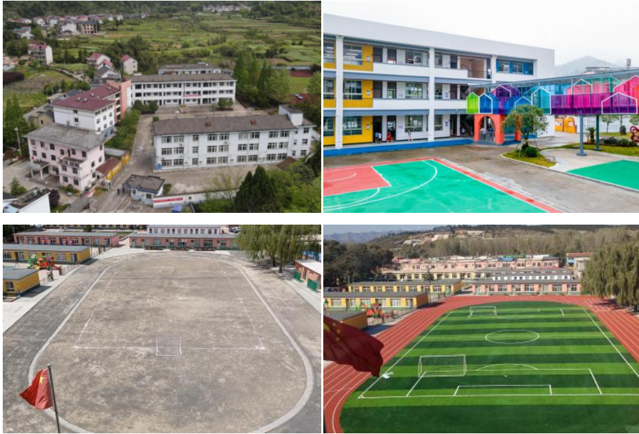
Photo: Xinchang Township Central Primary School supported by Hangzhou Branch (top) and Shanzuizi Township Central Primary School supported by Shenyang Branch (bottom) Comparison of school buildings and playgrounds before and after renovation
