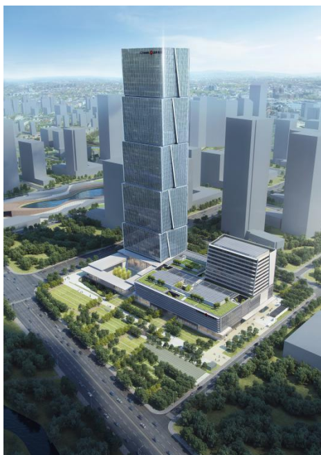
Photo: CZBank's headquarters building in Qianjiang Century City uses double glazed curtain walls, which
