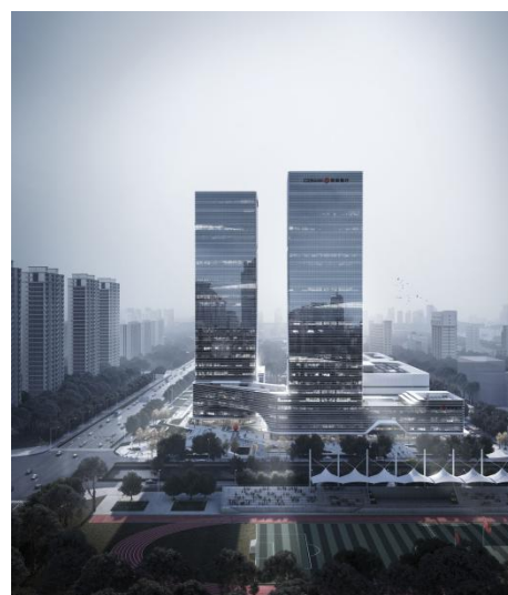
Photo: The Xi'an Research Center adopts a centralized solar hot water system and a rainwater recycling system. The former is expected to provide 6,108.69 m 3 of hot water per year, and the latter recycles rainwater to wash public areas and irrigate
