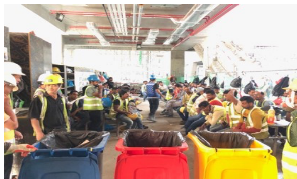
Segregation and recycling of waste on site
