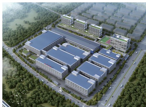
Ningbo Production Base
