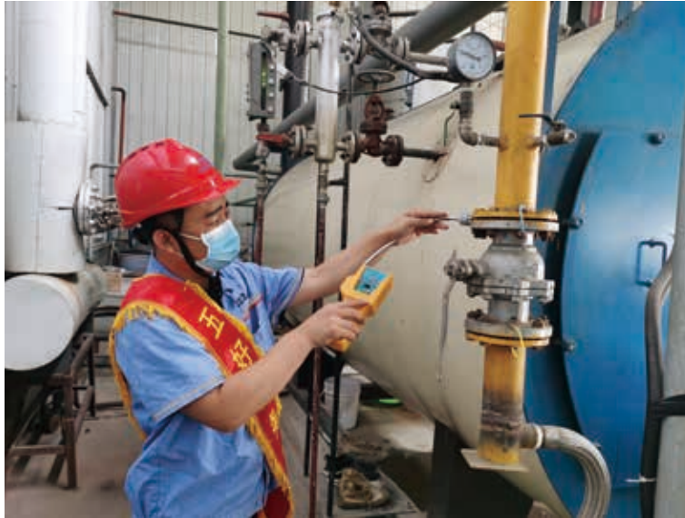
Safety examination by Tangshan Subsidiary Company 唐山公司安全檢修
