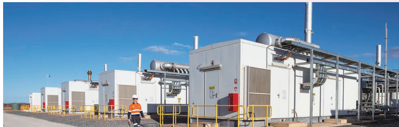
∞ The Agnew Hybrid Renewable Microgrid comprises wind, solar, gas and diesel generation and battery storage.
