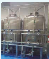
Purified water preparation system
