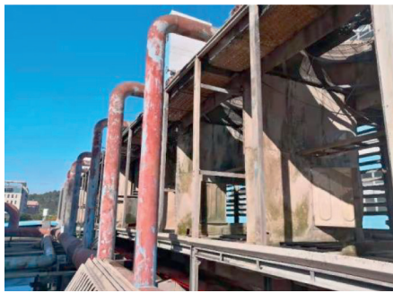
Before Transformation 改造前
