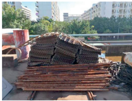
During Transformation 改造中
