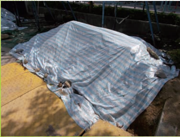
Cover the stockpile of dusty materials 覆蓋易生塵埃的物料堆
