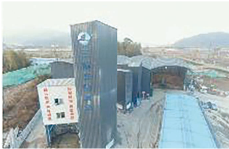
Enclosed mixing plant
