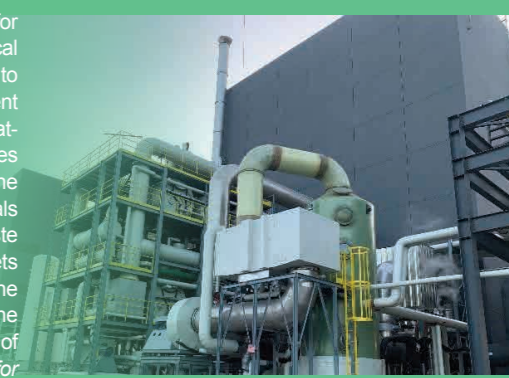
Picture note: Panorama of activated-carbon adsorption device
