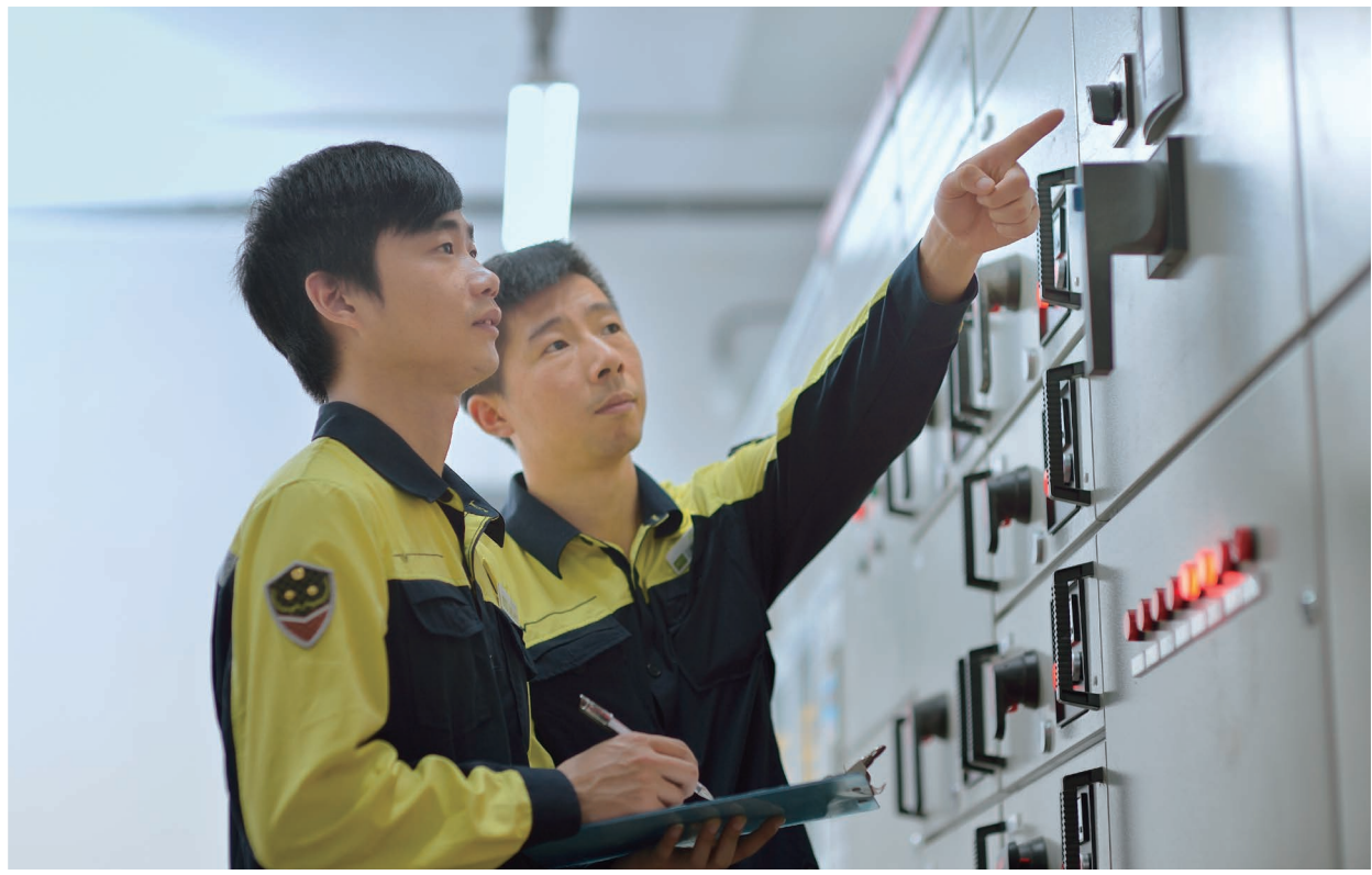
Onewo - Community Space Mechanical Room Maintenance & Inspection
