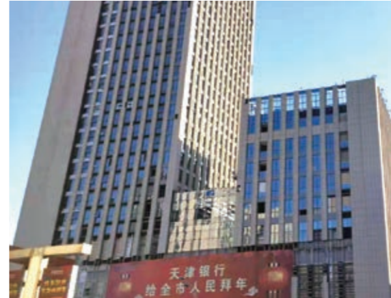
Back-office Operation Center (Under Construction)
