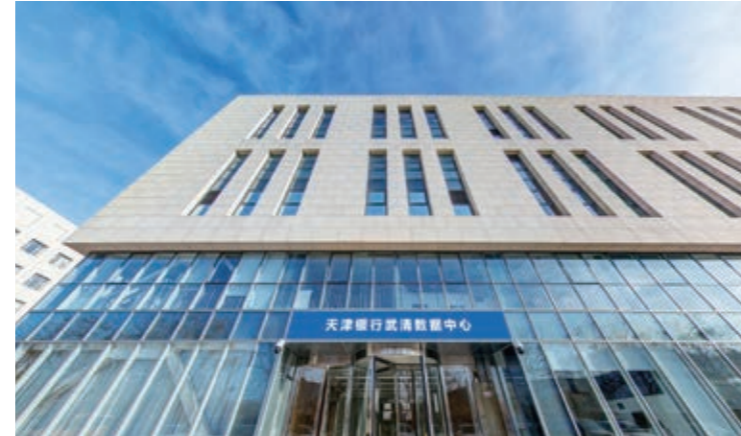
Wuqing Data Center
