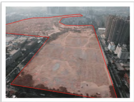
Before redevelopment 項目改造前
