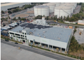
Waste Plastic Bottle Treatment Plant, EcoPark
