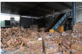
Waste Paper Recycling Centre, Sheung Shui
