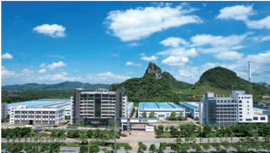
Rooftop distributed photovoltaic (DPV) project
