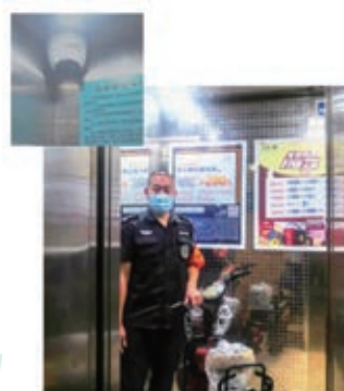
Battery Cars Barrier System in Elevators
