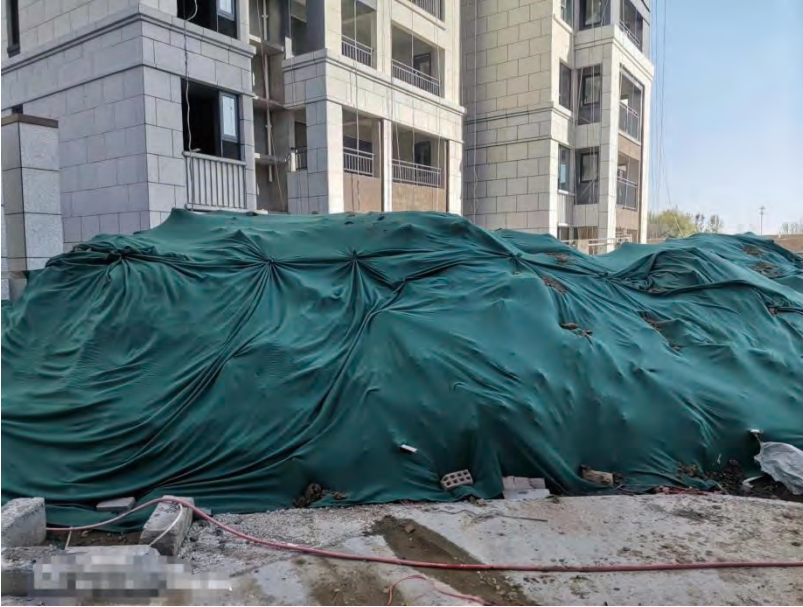
Covering exposed loess on site
