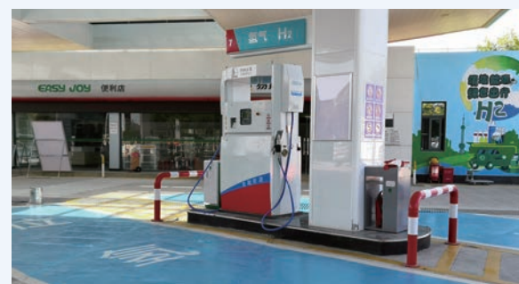
The largest hydrogen refueling stations with the highest filling pressure in China have been put into operation to serve the Olympics Winter Games
