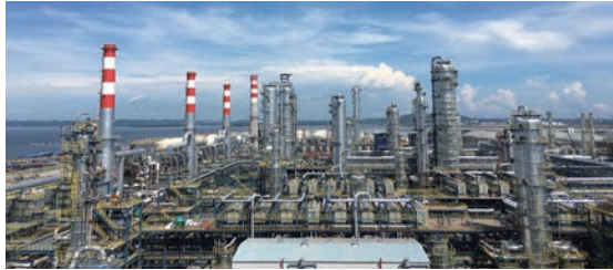
Hengyi (Brunei) PMB Petrochemical Project
