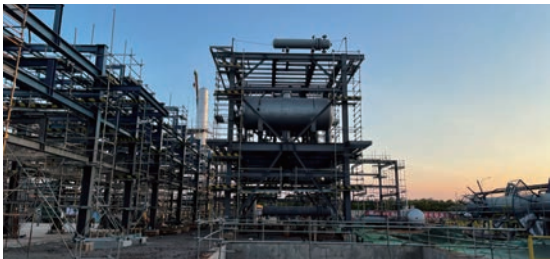
Green soiless construction
