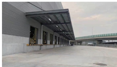
溫州樂清博科產業園 Wenzhou Yueqing Boke Industrial Park
