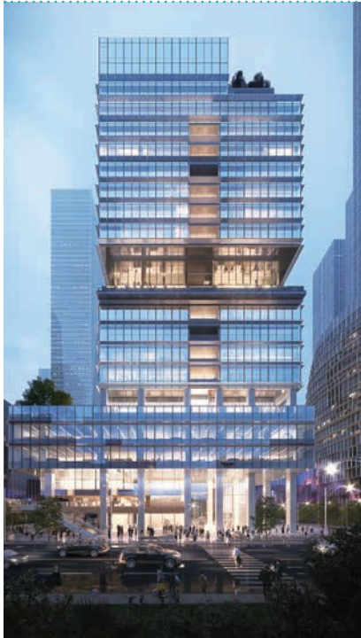
■ The Group's new headquarters in Houhai, Shenzhen
