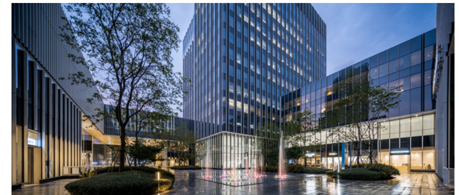
Green Automatic Sprinkler System and Reclaimed Water Reuse System
