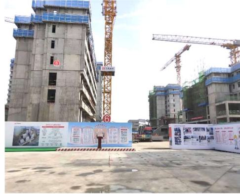
Hefei Branch supported the construction of talent apartments
