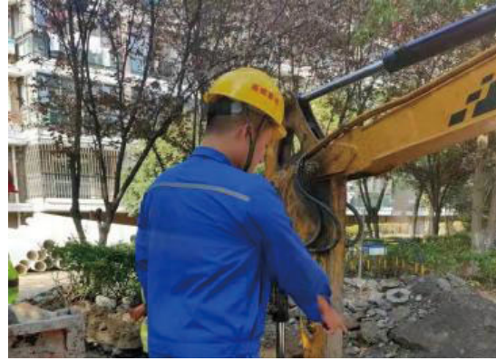
Photo: An on-site supervisor supervise the excavation work
