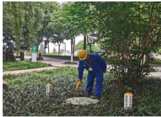
Photo: An inspector inspects the municipal pipeline network
