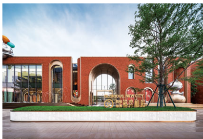
南寧福弈和庭 Nanning Fuyiheting Mansion
