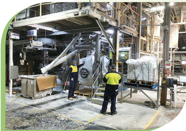
Cheetham's bulker station at the manufacturing facility in Price, Australia.
