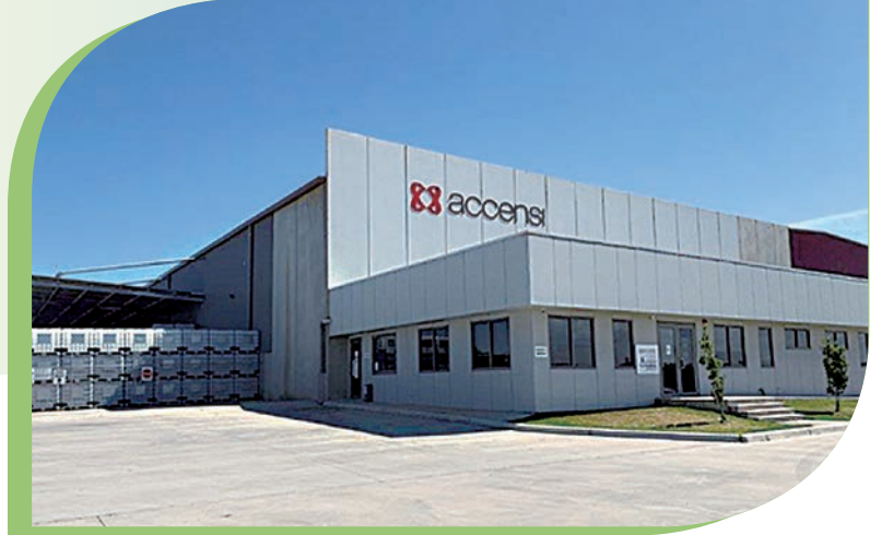
Accensi's manufacturing facility in Lara, Australia.
