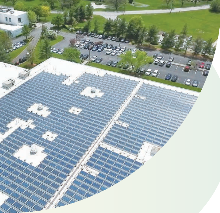
Solar panels installed at Vitaquest's headquarters.
