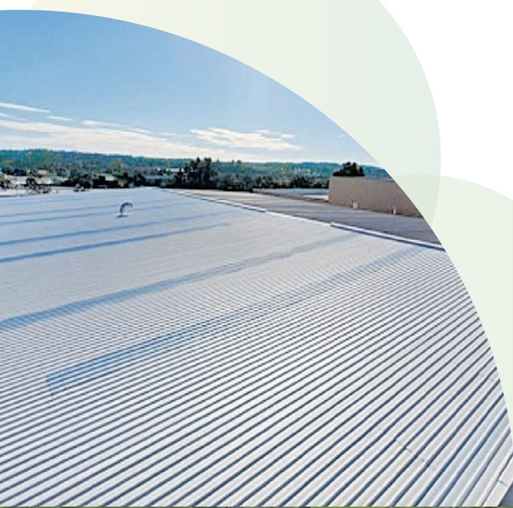
Lipa — Heat reflective paint (SkyCool) application at its warehouse.
