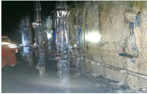
Picture: 110 Operation Approach for Mining Face at Zhaiyadi Coal Mine
