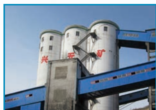
Xingwu Coal Mine 興無煤礦
