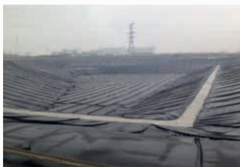
Figure 4 Anti – Seepage and Leakage Improvement Work at Yancheng NUHF
