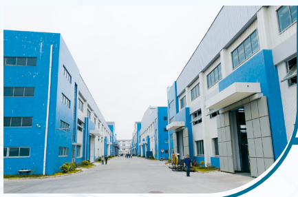
A corner of the plant of Fong's National Engineering (Guangdong)
