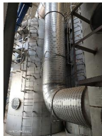
Spraying Tower for handling of paint exhaust
