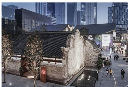
Old temple protection and renovation
