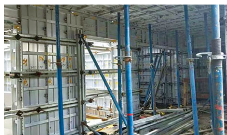
Prefabricated reusable building components on construction site
