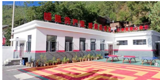
兰坪县北甸小学食堂 Beidian Primary School Canteen, Lanping County
