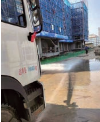
Watering for dust control 水車灑水抑塵
