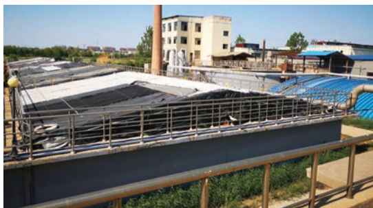
Sewerage treatment station
