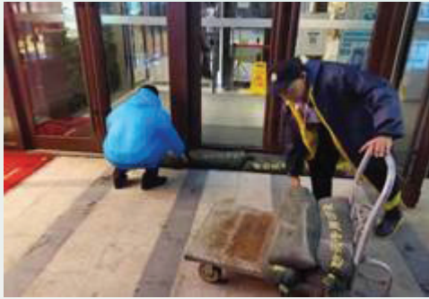
Sealing doors with sandbags
