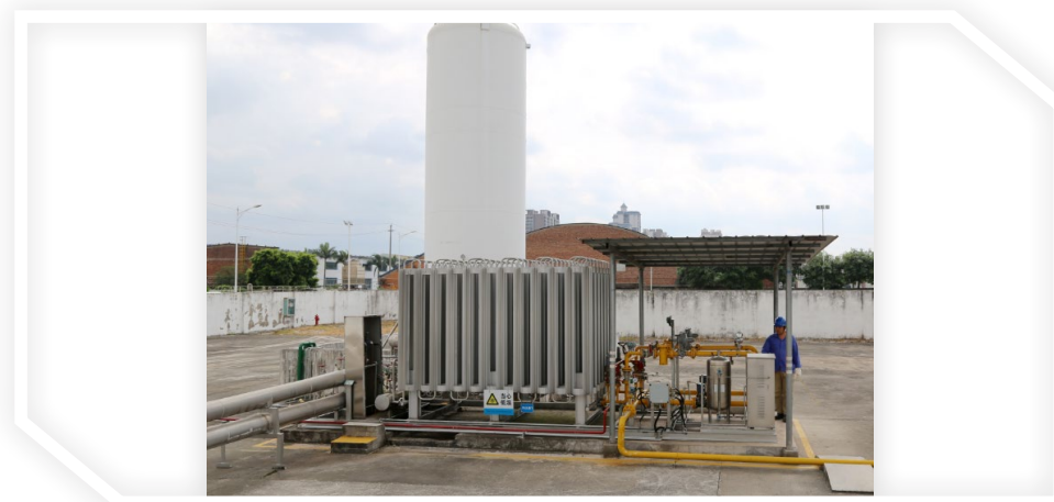
Inspections on eliminating major hazard sources 消除重大危險源巡檢
