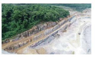
Jiangxi Ya Dong implemented presplit blasting of finished slopes, having maintained the integrity and stability of rock mass
