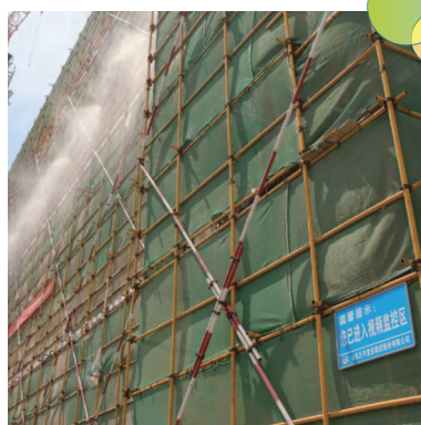
腳手架噴霧降塵降低揚塵措施
