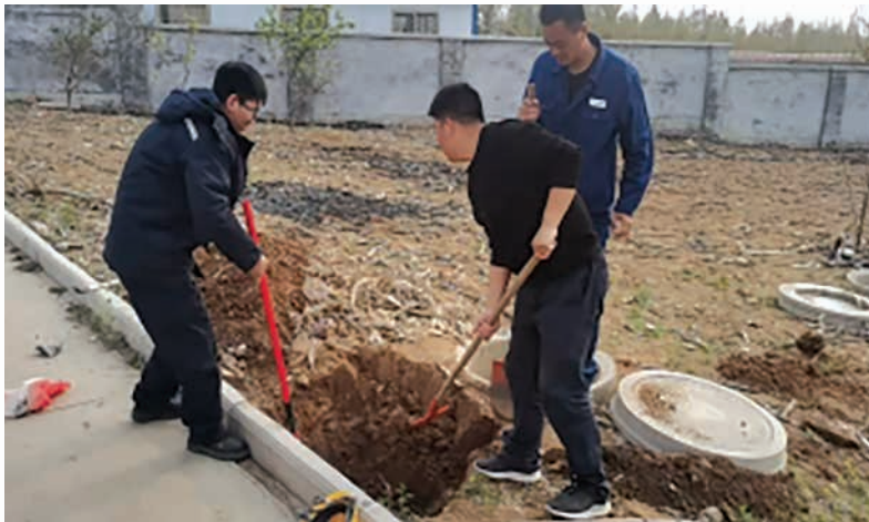
Repair for the sewage system of Shandong Loude Power Station
