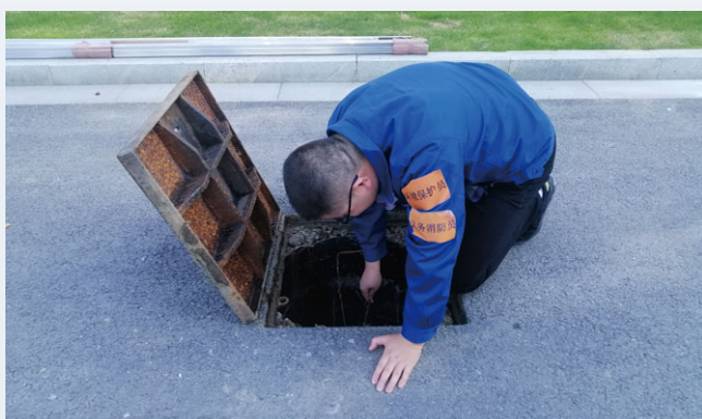
Daily environmental fire hazard inspection 日常環境消防隱患檢查
