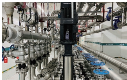
Water pump house after upgrading
