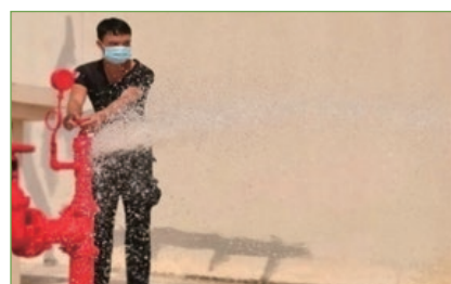
💧 Waterproof test of fire hydrant on the roof
