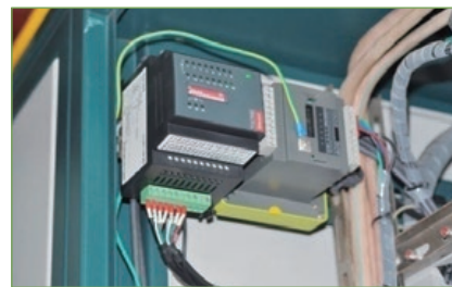
💧 EBA system for monitoring operation of equipment in the pump room
