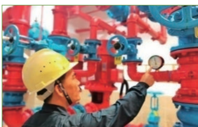
💧 Inspection of spray pipes
