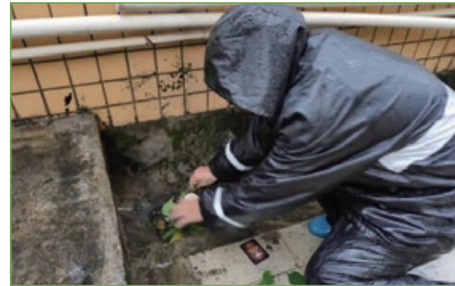
💧 Dredging of drainage network
