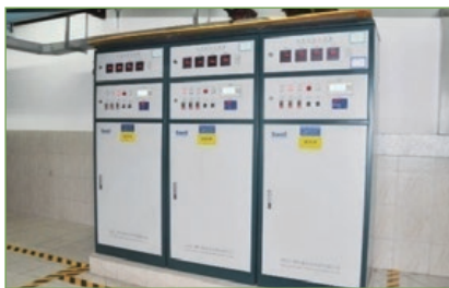
💧 EBA system for monitoring operation of equipment in the pump room
