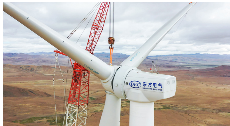
◀ 東方電氣為世界最高海拔風電場——西藏措美縣哲古分散式風電項目提供的 5 台 2.X-131 型永磁直驅超高海拔風電機組全容量並網發電 5 DEC 2.X-131 permanent magnetic direct drive wind turbines applicable to regions of ultra-high attitude were put into grid-connected power generation at full capacity in the world's highest-altitude wind power project—a distributed wind farm located at Zhegu, Cuomei County, Tibet
